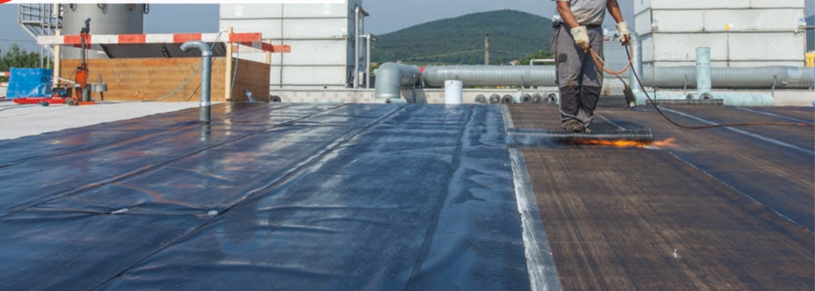
Seam welding with hand welder
